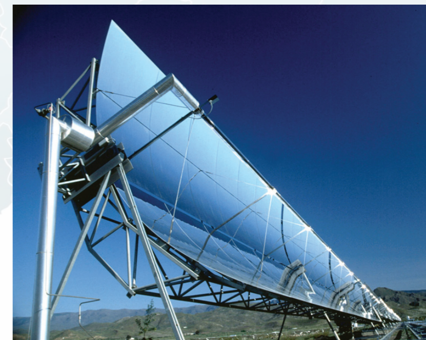
Detail of parabolic mirror at the Archimede solar plant
