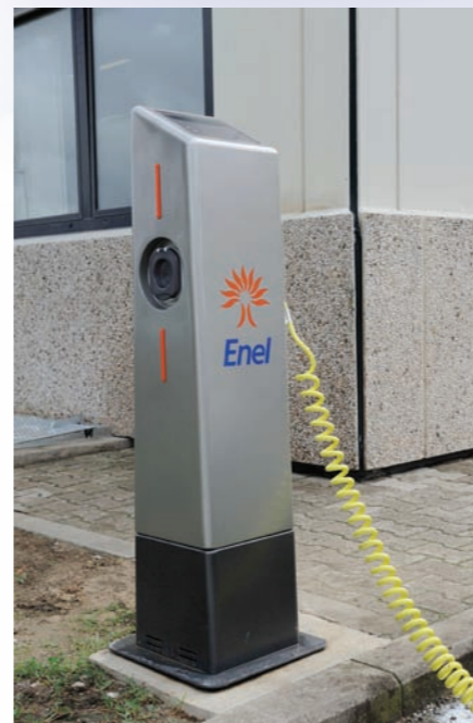
Enel E-mobility recharging column
