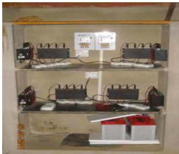
**Figure 4.21: Solar central charging station for detachable batteries.** (Source: Selco)
